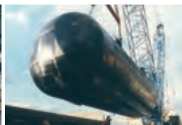
Tanks: External coating of tanks for installation in a chemical plant
