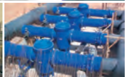
Great Man-Made-River Project, Libya: Water supply distribution unit protected with PROTEGOL®UR 32-55
