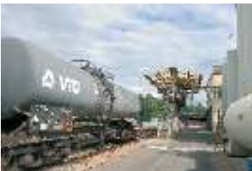
Filling station for tank wagons and street tank cars
